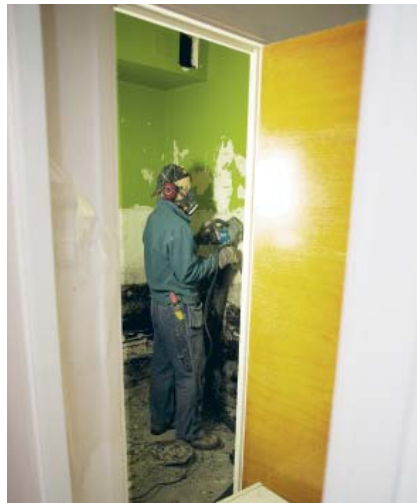
Grinding machine with a suction casing and the aircleaner DC AirCube as back-up.
