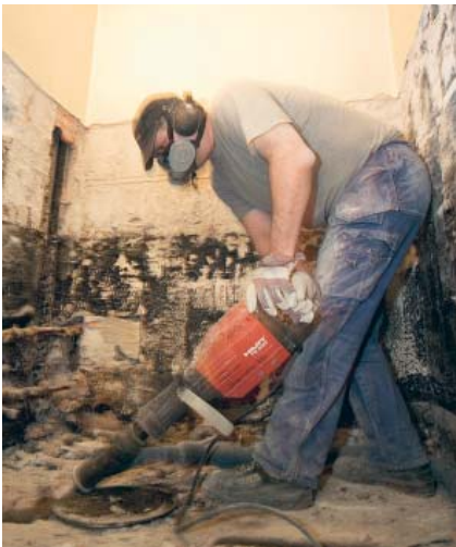
Hilti 905 with a suction casing from Dustcontrol.
