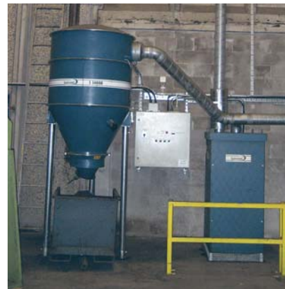
Hot air from the central unit is pumped back into the premises in the winter to save heating expenses.
